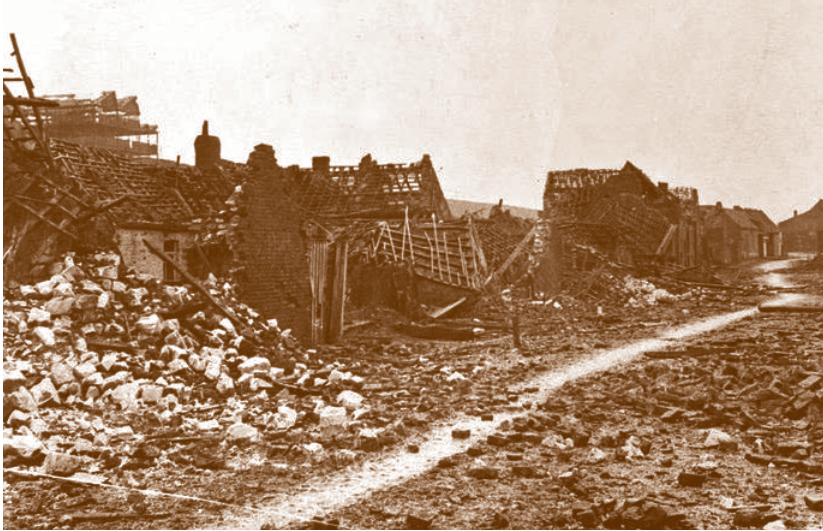
Ruins in the church quarter of Loos, 24th November 1915. (c) IWM (Q 58151)
