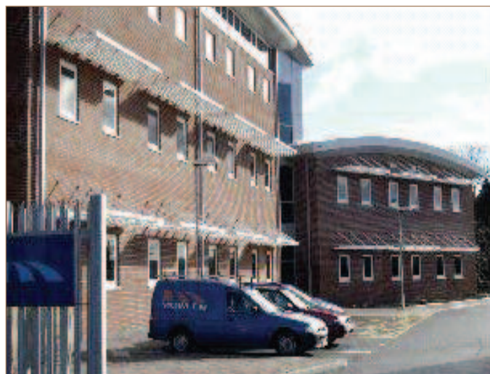
The New Scientific Support Unit at South Wales Police Headquarters in Bridgend
